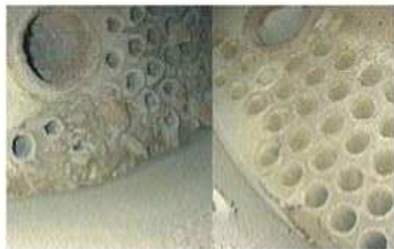
Tubes before and after cleaning with an APCS
